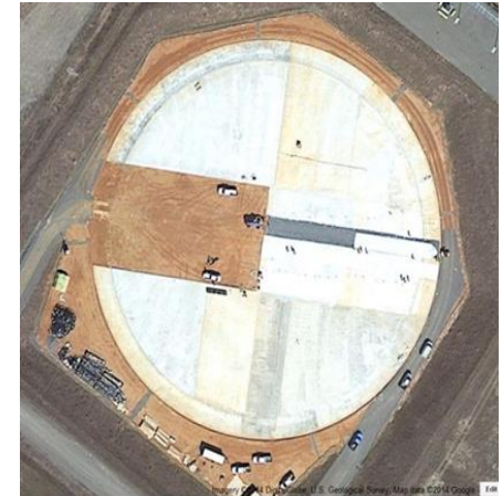
Much Larger Circular Disposal Structures (currently under construction)
