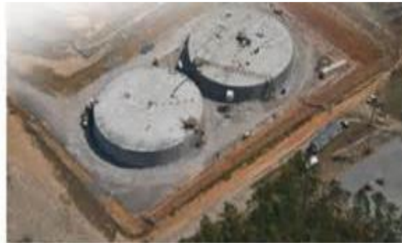
Circular Disposal Structures
