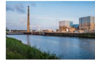
Brunswick Nuclear Plant Southport, N.C.
