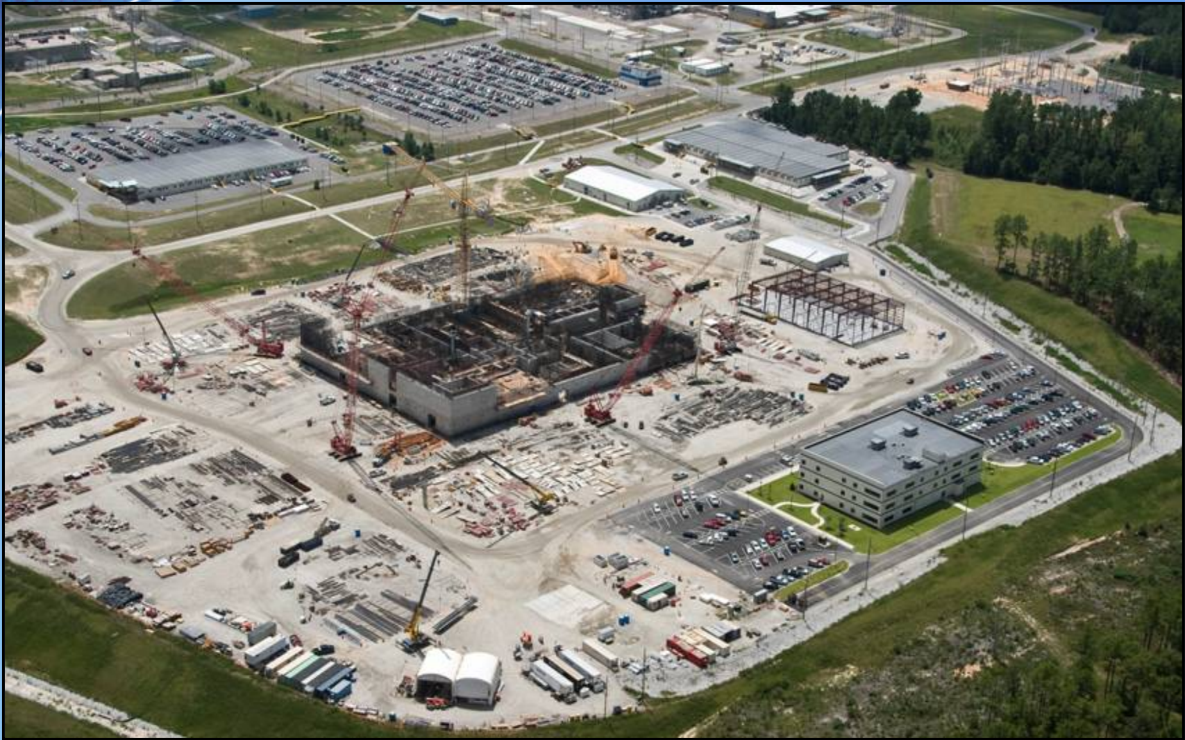
MOX Construction Site - August 2009
