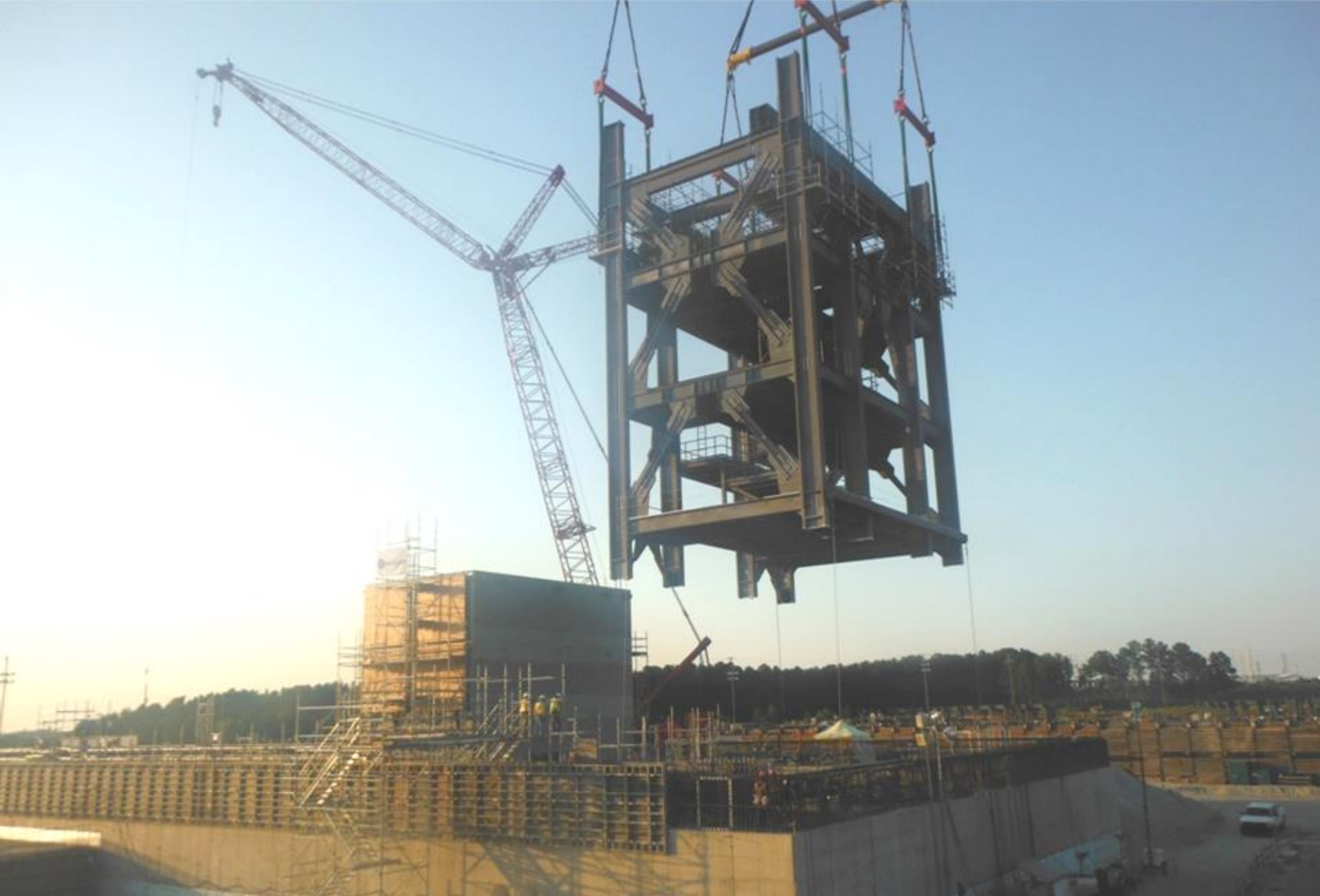
Unit 2 Turbine Building – CH80 Steel Set
