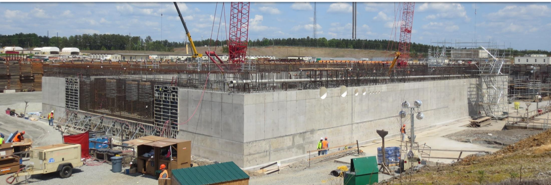
Unit 2 Turbine Building
